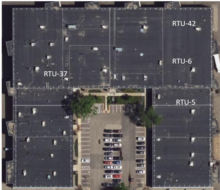
Figure 30. Site 3 aerial view of RTUs
