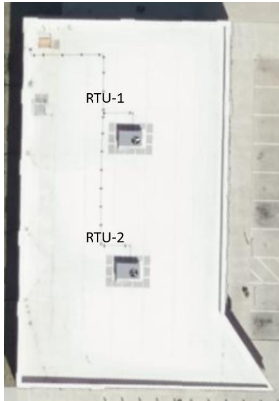
Figure 29. Site 2 aerial view of RTUs
