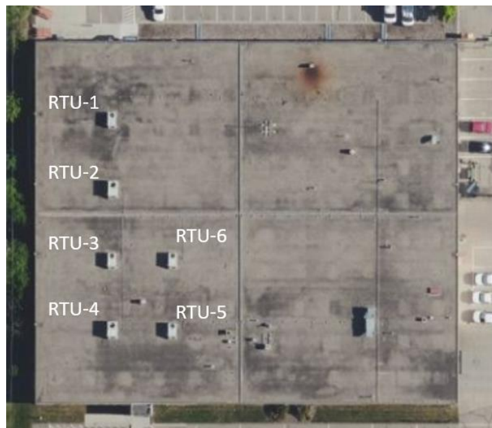
Figure 28. Site 1 aerial view of RTUs
