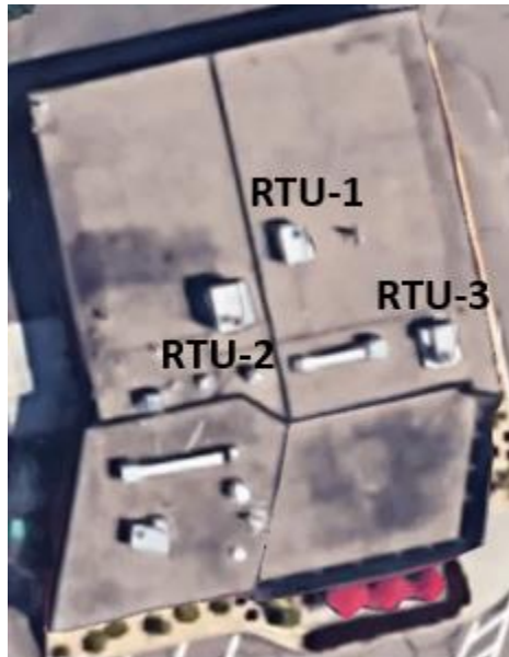
Figure 32. Site 6 aerial view of RTUs
